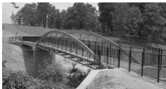
The Lisbon Bridge Restored as entrance to the Columbiana County Fairgrounds
