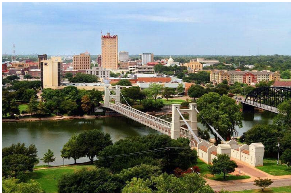
Waco Suspension Bridge. Photo: Nathan Holth, HistoricBridges.org .
