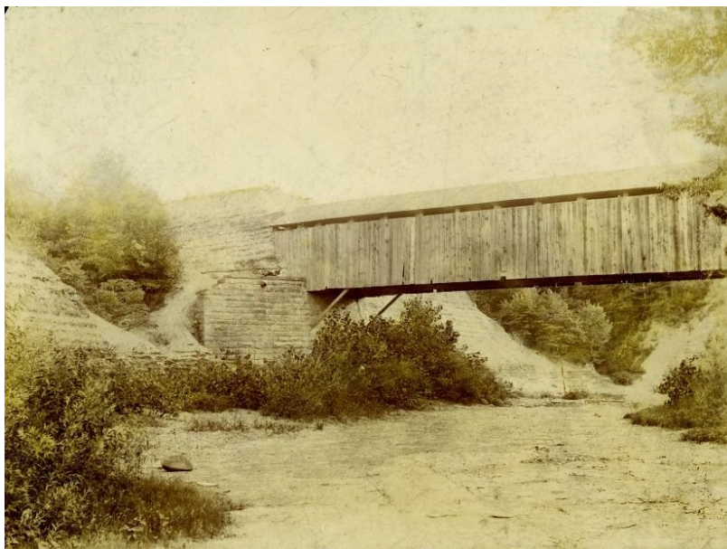
The shale cliffs at the site dominate the background of the 1858 Myers Mill Bridge. Sherman used a very low arch for his Burr trusses, so the ends of the arch on the abutment are hidden behind siding. Additional end braces—not the arches—had also been added to support the end. By the late-19 th -century date of this photo, the two coats of white paint specified for the siding had long before weathered away. Credit: Delaware County Historical Society
