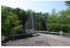
ple, with the only alteration being new floor beams, open-grid steel flooring, and new guardrails. Even with the addition of newer "high-impact" guardrails, the county engineer was careful to preserve the original lattice railings.
