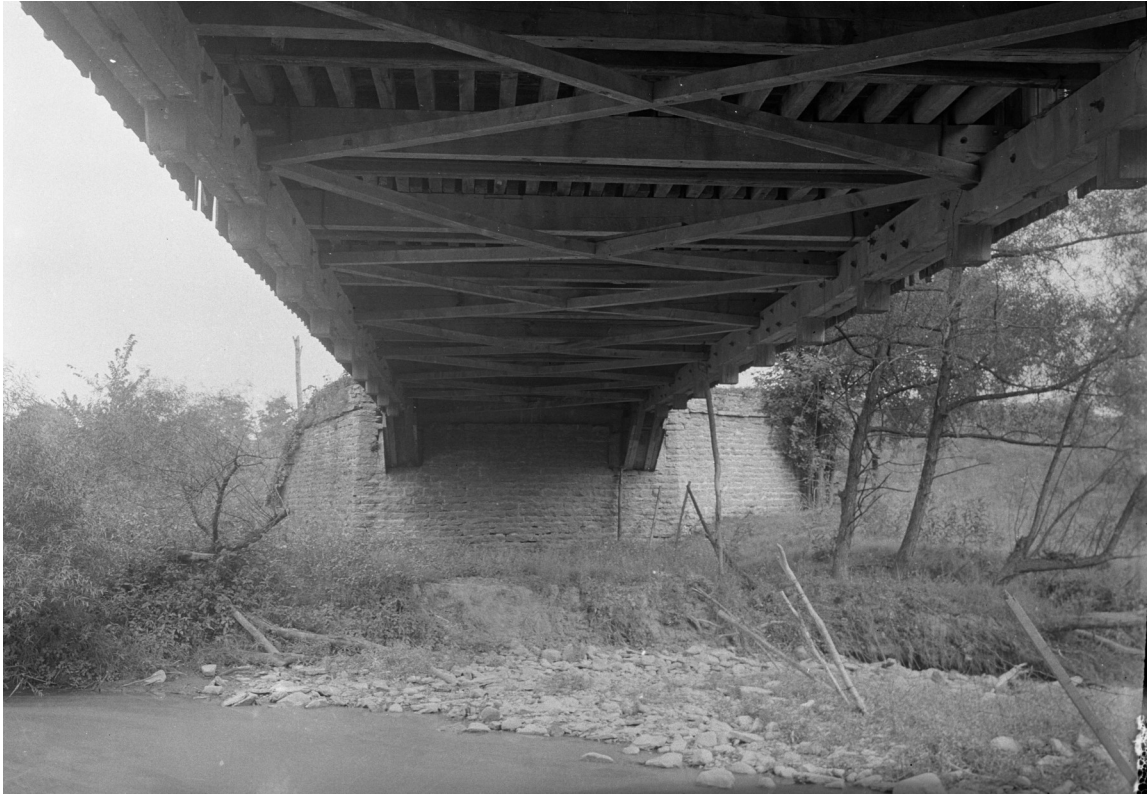
The massive western abutment on the Fairfield Pike location indicates that the county had major concerns about flash flooding at the new location.
