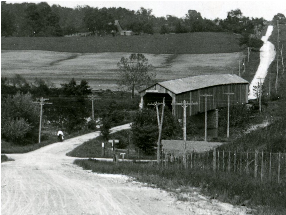
The Scioto River Bridge in Delaware County's Scioto Township was built in 1864, but most of the original two coats of white paint had weathered away when it was photographed at the turn of the 20 th century. More importantly, however, the original camber was still apparent Ohio History Connection, SC 1156
