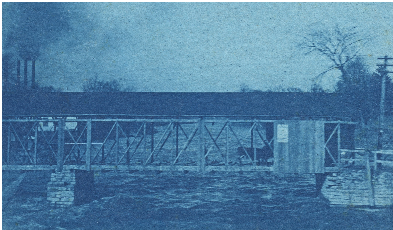
Prospect, Ohio, resident T. E. Howald photographed Delaware County's Stratford Bridge as he sped by on the interurban bridge, the piers from which still stand in the Olentangy River. The photo has to postdate 1903, when the interurban began operating. Todd Clark Collection
