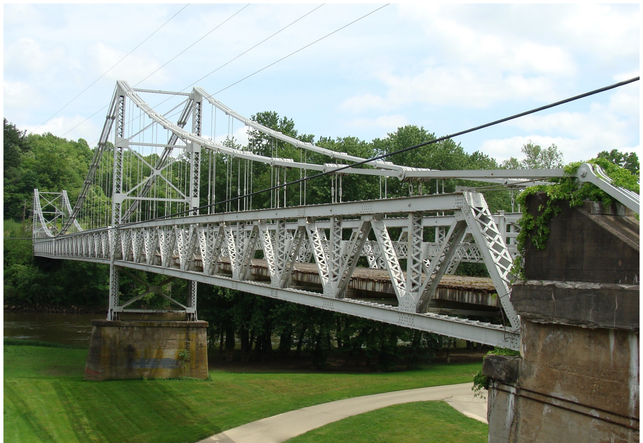
Dresden Suspension Bridge over the Muskingum River - Photo by David Simmons
