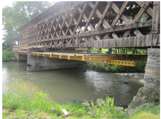
Mull Covered Bridge, Sandusky County During Construction
