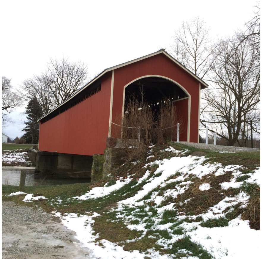
With funding facilitated through the Sandusky County Commissioners and county park district, who owns the bridge, the 2015 Mull Road Covered Bridge project replaced the old siding and roof. (Photo by David Simmons)
