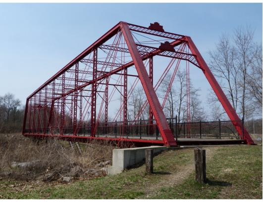
exhibit there, along **Charlotte Highway Bridge, Calhoun County Historic Bridge Park** with an 1892 stone arch still used by Amtrak. One of the most impressive is the 177-foot doubleintersection Pratt through truss, the former Charlotte Highway Bridge, built in 1886 by the Buckeye Bridge and Iron Works of Cleveland, Ohio.
