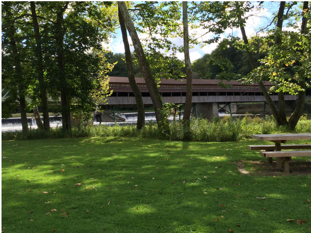
Harpersfield Covered Bridge photo by Elma Lee Moore
